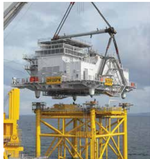
Foundation for substation at Gwynt y Môr
